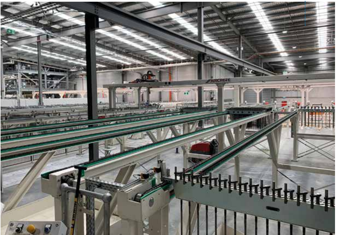
Fig. 3: Multiple handling devices are required in an automated reinforcement area
