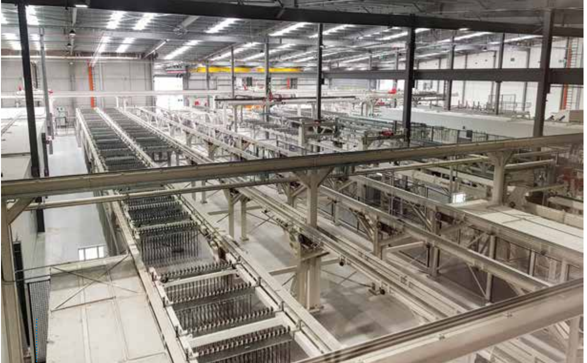
Fig. 2: An overview of the automated reinforcement area
