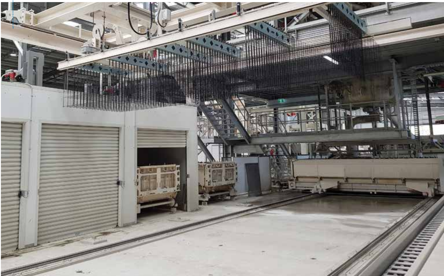
Fig. 7: The reinforcement frame as it travels to be placed in the mould
