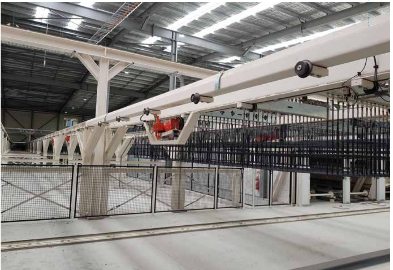
Fig. 6: Reinforcement is automatically assembled on the needles of the reinforcement frames
