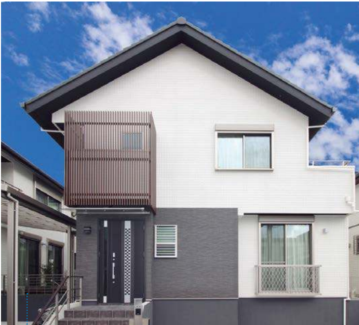
Fig. 5: AAC cladding panels provides a durable insulation layer on outer walls with esthetical appearances
