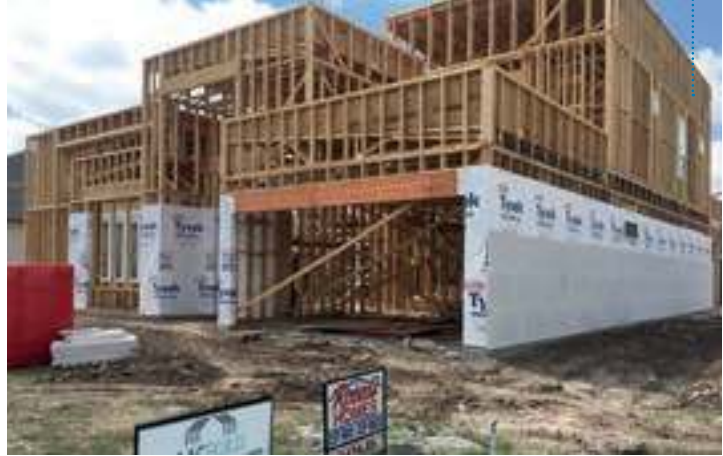
Fig. 3: The US buildings market is highly dominated with wood-frame construction, where AAC panels are an ideal material for resilient buildings
