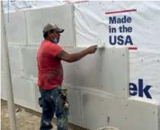
Fig. 2: Thin lightweight AAC panels usage in the form of cladding systems from AAC Build in Texas
