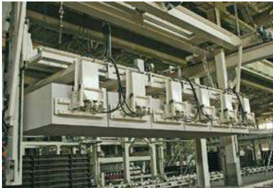
Fig. 12 The unloading crane grabs the full length of the cake and transfers the entire cake from the frame onto the pallet table.
