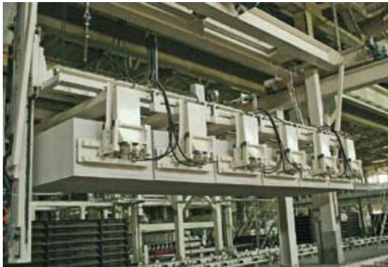
Fig. 12 The unloading crane grabs the full length of the cake and transfers the entire cake from the frame onto the pallet table.
