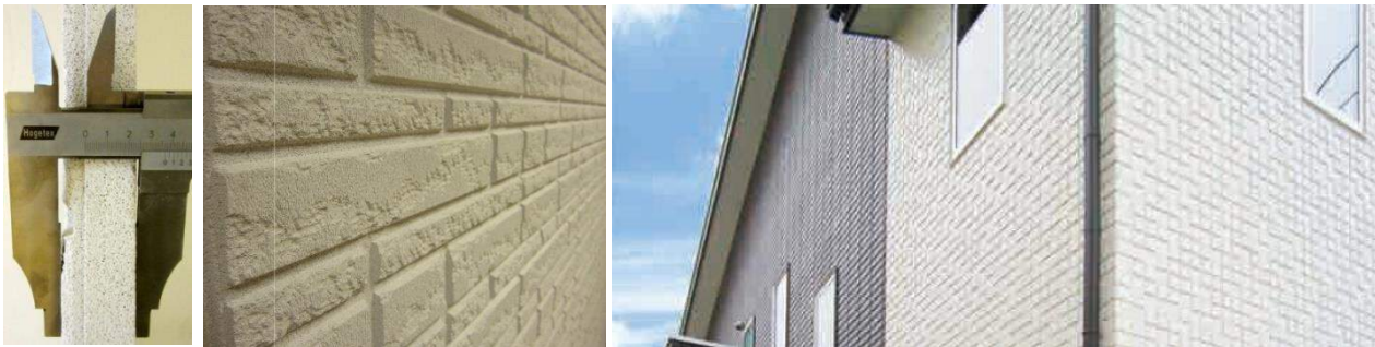
Fig. 3 Cladding panels application (L x W x H – 2m x 0.6m x 35 mm)
