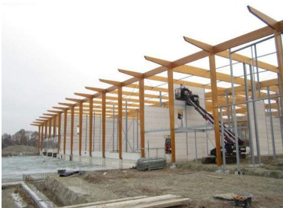
Fig.2 Industrial warehouses – AAC Panels used on the wooden and steel structures.
