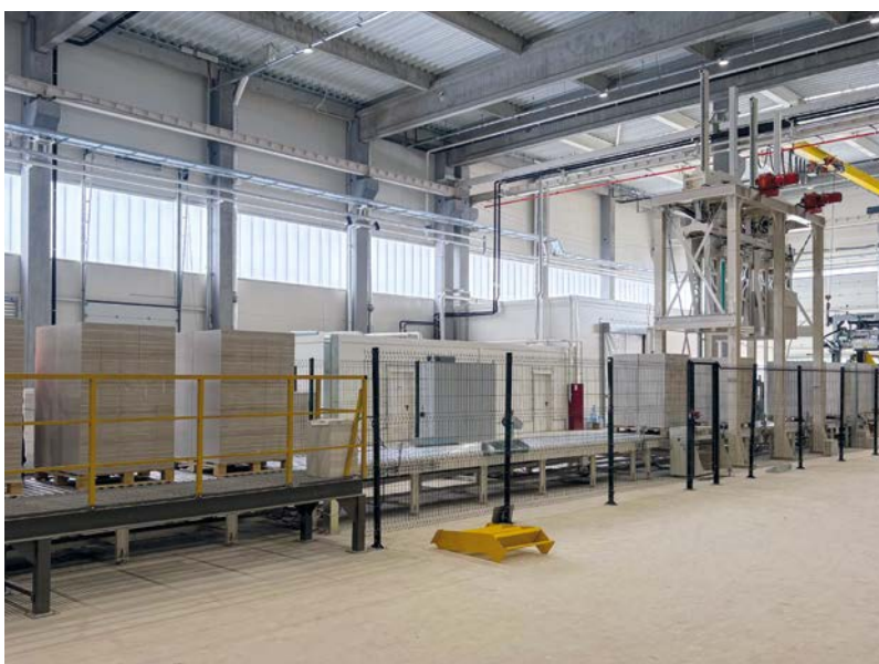
Fig. 9: Unloading line featuring automated pack configuration for flexible pallet height and product sorting.
